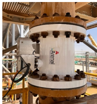
Figure 2.2: Arenal Ultrasonic Density Meter in Pipeline
