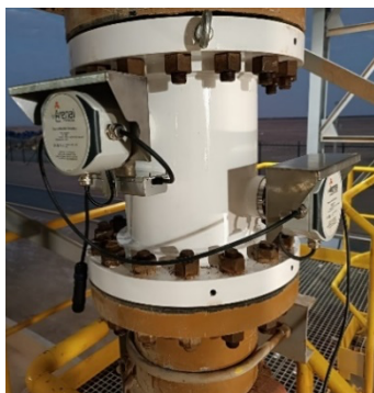
Figure 2.1: Arenal Ultrasonic Density Meter in Pipeline
